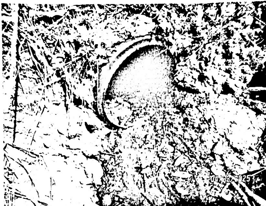
Photo 17. View of an HDPE pipe observed on the downstream side of the spillway; however, not visible along the upstream headwall structure. however, appeared to be leaking.
